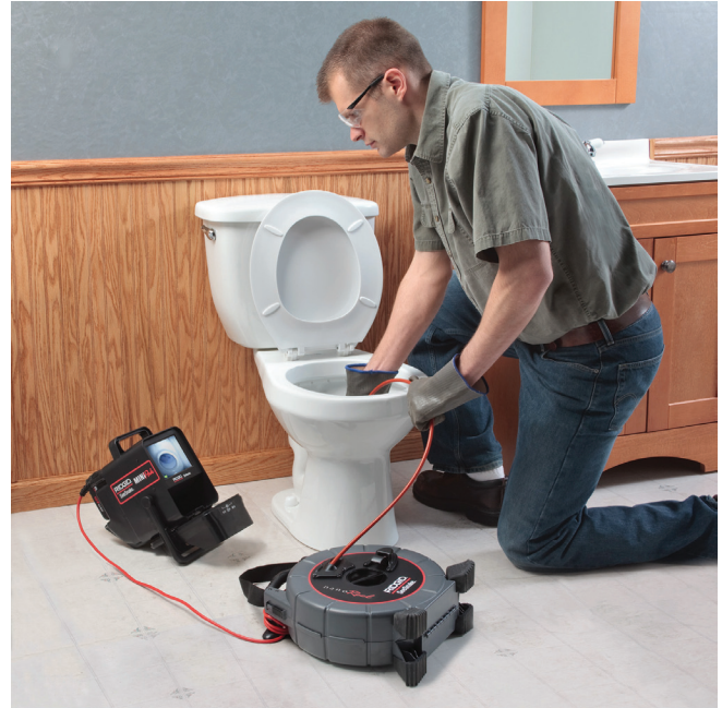
Figure 14 – Performing an Inspection
